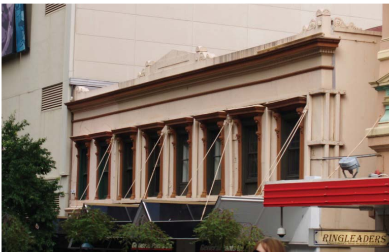
Figure 19-9 William Cairncross Building
